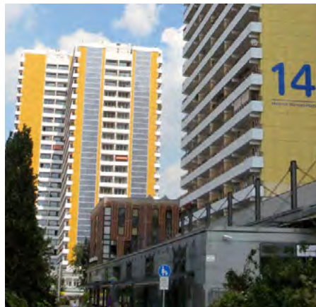
Solar wall tower retrofit, Berlin, Germany, 2009
